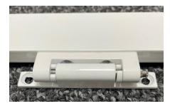
At this point you can't see the holes to mark them so hold the hinge firmly against the frame and
