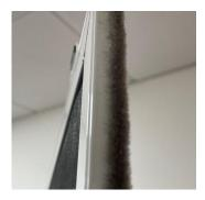
• Now repeat with the second screen but this time put the pile to the back of the frame i.e. closest edge to your door frame.
